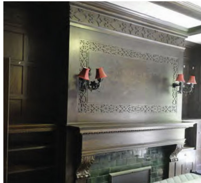
EXISTING MILLWORK RELOCATED FROM CLAVERLY SUITE #9
